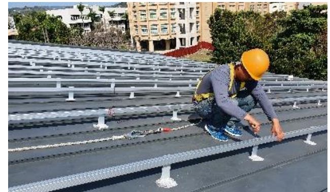
▲ Solar Panel Installation Works
