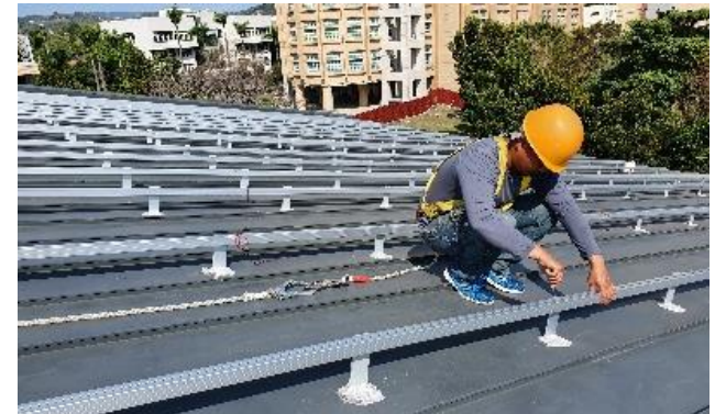
▲ Solar Panel Installation Works
