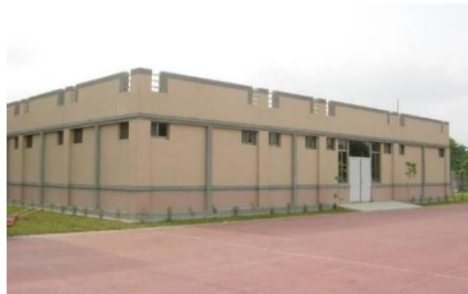
▲ Wastewater Treatment Plant
